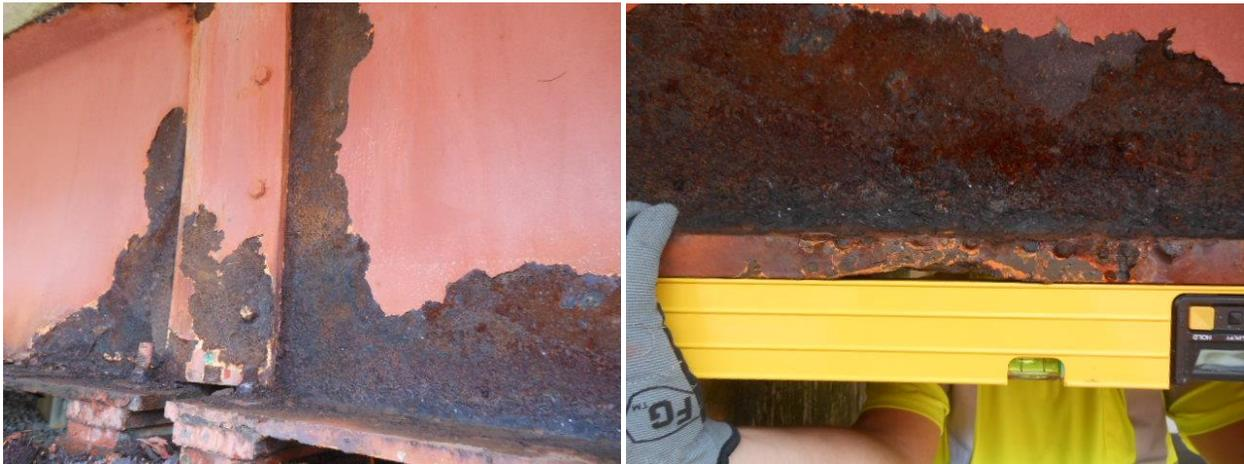
**Figure 15—Superstructure Deterioration: (a) Deterioration in Web and Bottom Flange
