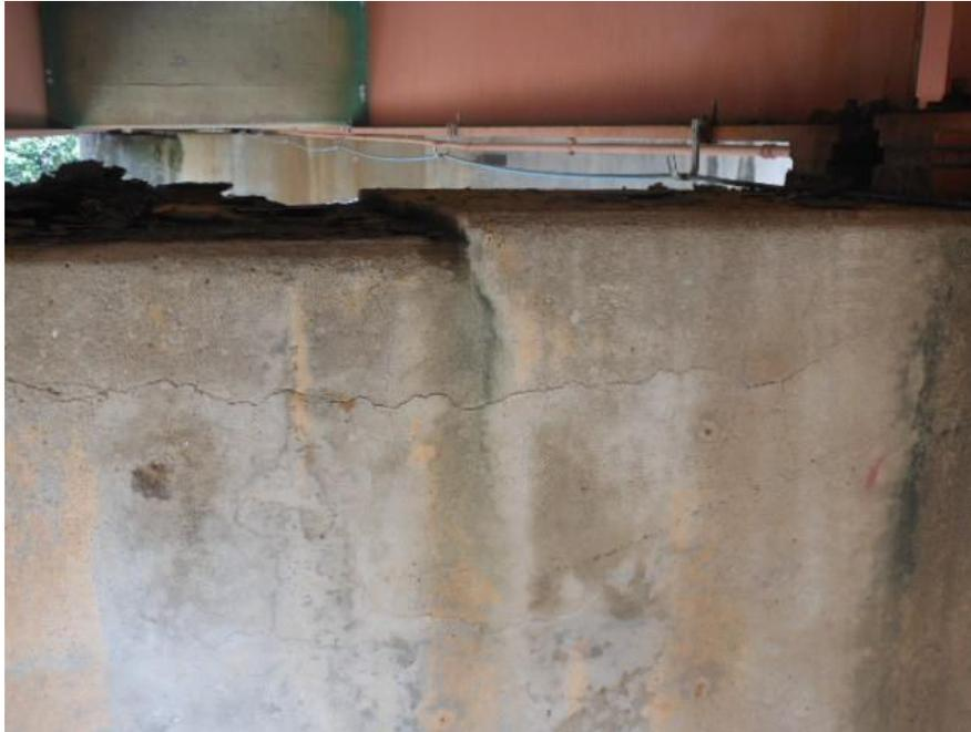
**Figure 16—Horizontal Crack in Bent Cap [GDOT, 2017]**
