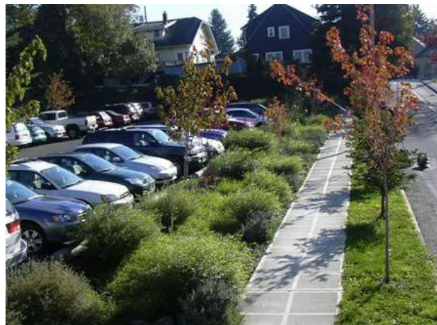
Figure 3.9 Swales on parking lots can absorb runoff from the large amount of impervious lot surface
