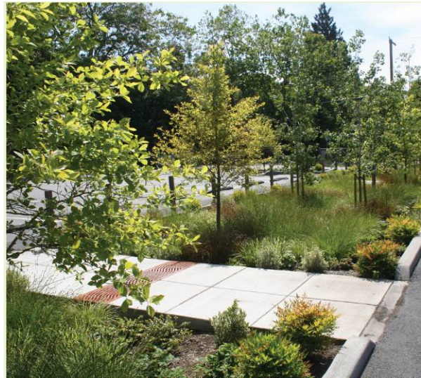
Figure 3.11 A large rain garden implemented in a parking lot space (source: Nevue Ngan Associates 2011)
