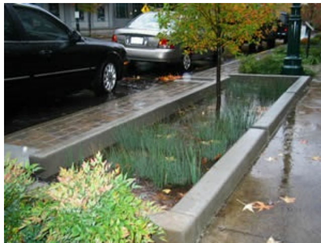
Figure 3.5 Stormwater planter with curb cut on 12th Avenue Green Street Project in Portland, OR (Source: www.portlandoregon.gov )
