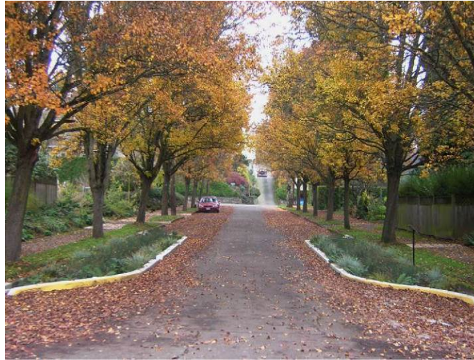
Figure 3.2 Green Street Project (North East Siskiyou Street) in Portland, OR with stormwater curb extensions (Source: City of Portland 2014 Stormwater Management Manual)
