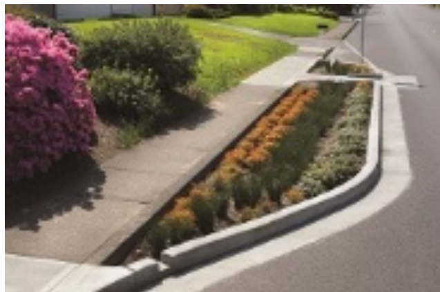
Figure 3.10 This street incorporates an angled stormwater curb extension, providing an ADA-compliant ramp for pedestrian access to the sidewalk (source: City of Portland, OR)
