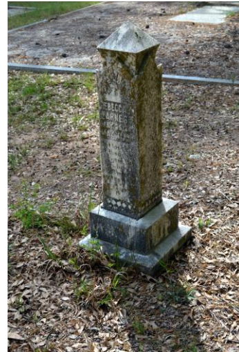
Figure 101. A grave marker in the Swords Community Cemetery with moss buildup and general soiling (Riley)
