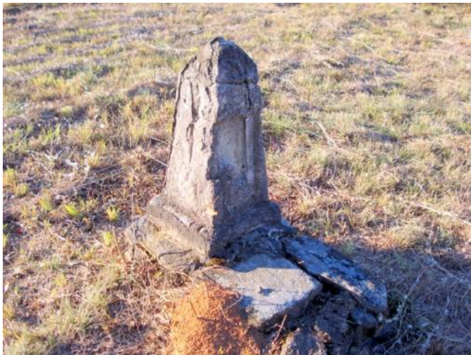
Figure 69. Precipitation and possible freeze-thaw damage on a marker at the Ponder Cemetery (Riley)
