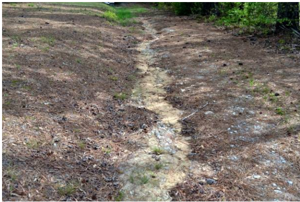
Figure 82. Runoff and vehicle erosion on the roadway in the Swords Community Cemetery (Riley)
