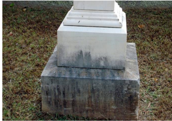
Figure 79. Damage to a marker in the Old Madison Cemetery from a riding mower and an edger (Riley)
