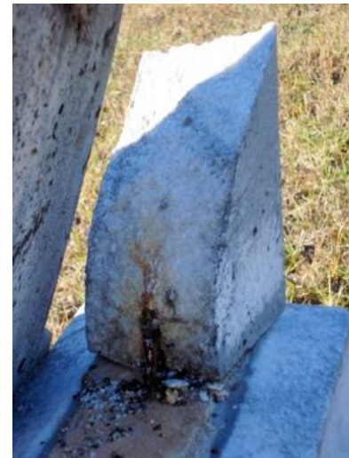
Figure 70. Damage from iron jacking on a grave marker in the Prospect Methodist Church Cemetery (Riley)
