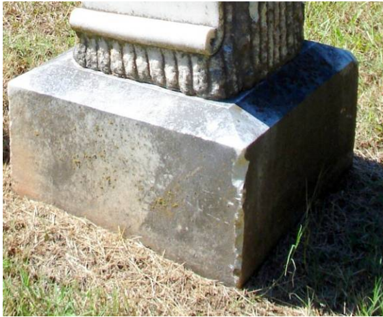
Figure 78. Damage to a marker in the New Cemetery from a riding mower (Riley)
