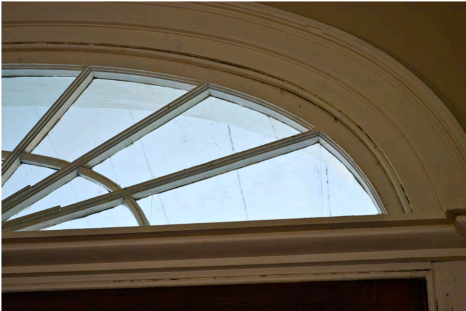
Figure 60, Joinery of Glass Panes Seen in Faint Vertical Lines of the Terrell House's Fanlight, Present Day
