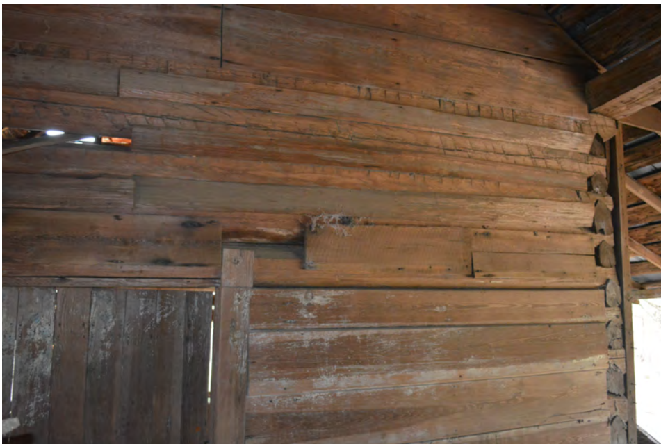
Figure 83, Boards Covering Gaps in the Interior Log Wall of the Saunders House's Dogtrot, Present Day
