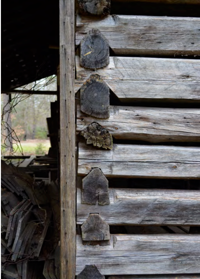
Figure 82, Detail of Log Joinery on the Saunders House, Present Day
