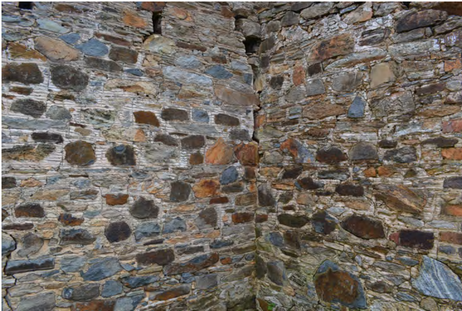
Figure 111, Detail of Coursed Rubble Former Outbuilding at Oakland Plantation, Present Day
