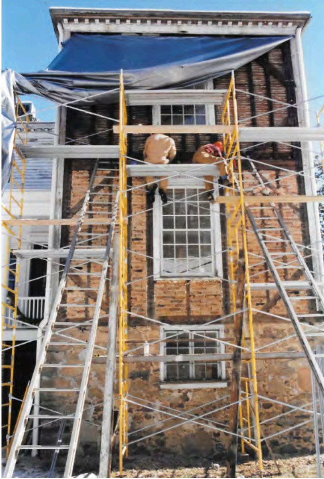
Figure 61, Brick Nogging in the Terrell House Revealed During Restoration in the 1990s
