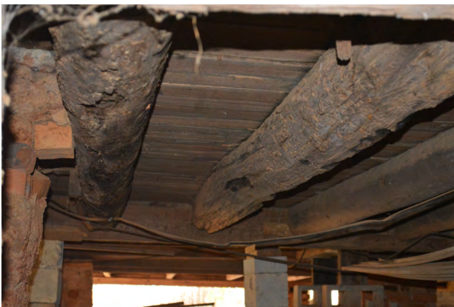
Figure 79, Hand-Hewn Timbers on the Underside of House in Southwestern Hancock County, Present Day
