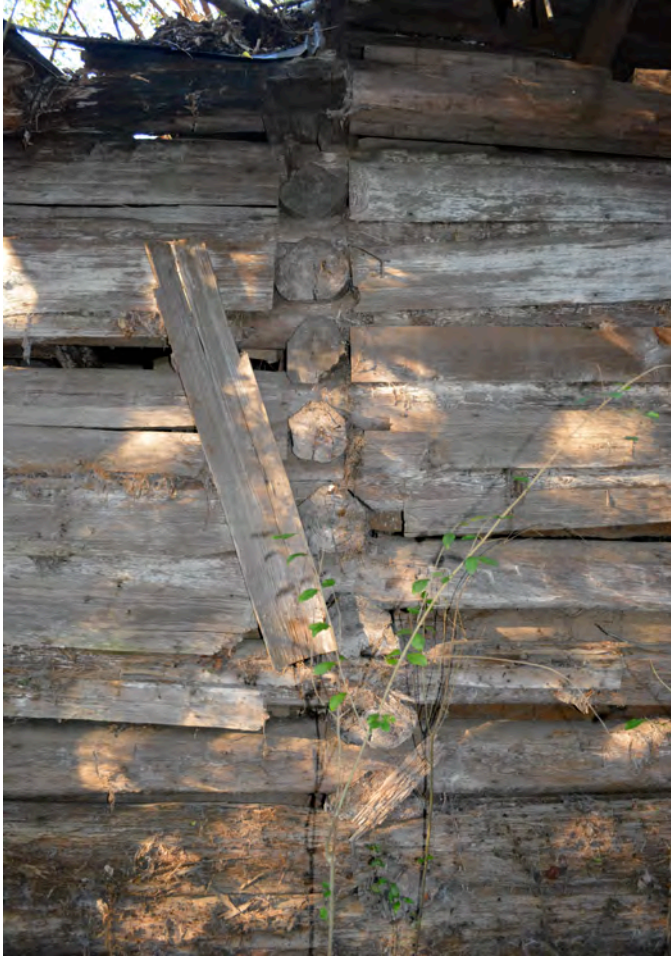
Figure 114, Detail of Notching on the Amos House, Present Day
