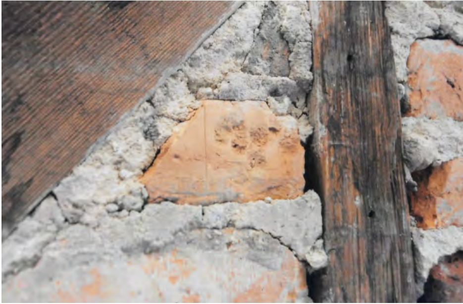
Figure 65, Fingerprints on Brick Nogging in the Terrell House Revealed in the 1990s
