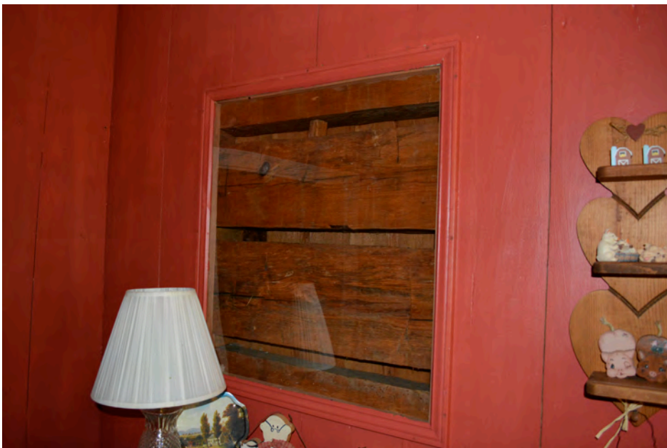
Figure 129, Reveal Incorporated into the Interior Wall of the Copeland House, Present Day
