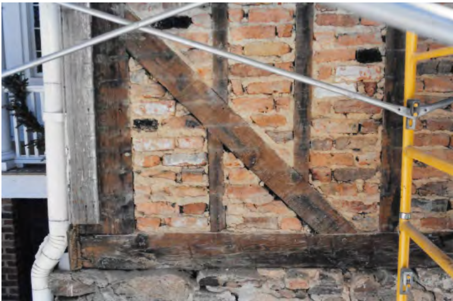
Figure 64, Detail of Brick Nogging in the Terrell House Revealed in the 1990s
