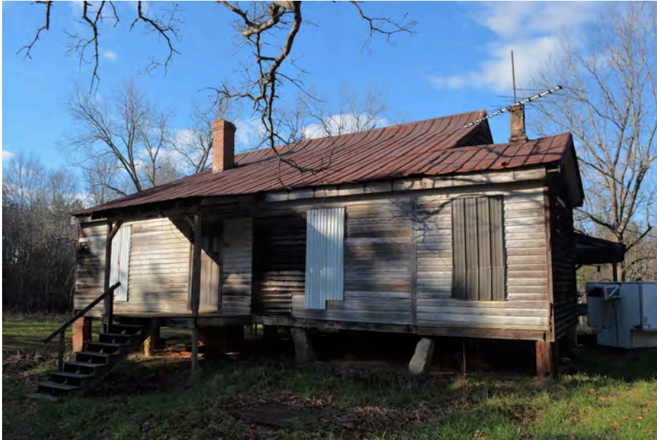
Figure 100, Original House, Showing Unsupported Section, Present Day
