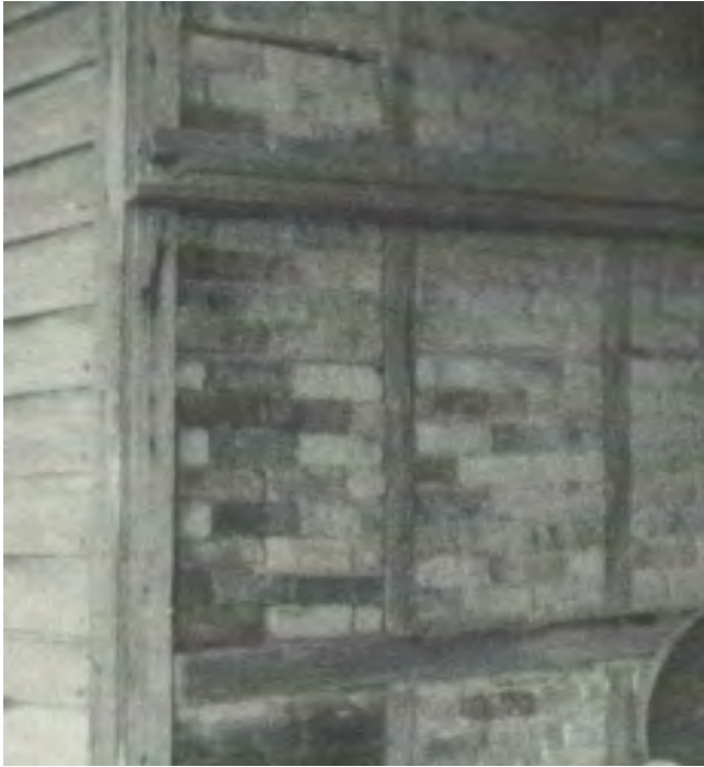
Figure 63, Detail of Brick Nogging in the John Roe House in an Undated Photograph
