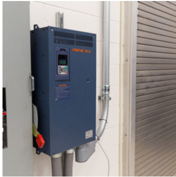
Figure 2.3: Front panel of variable frequency drive
