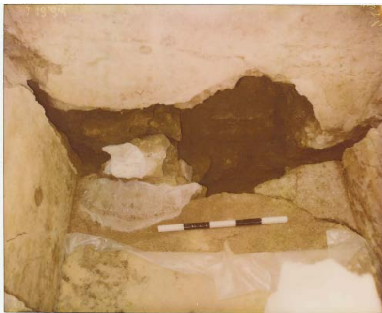
Figure 12: Crack in floor and south wall of Mini-Columbarium, looking south. Image Source: UGA Yasmina Excavation Archive
