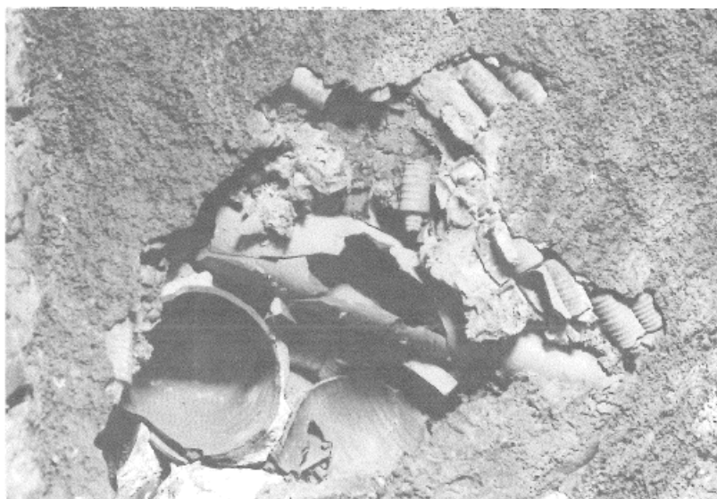
Figure 27: Vaulting tube framework with broken amphorae caementa above, Maison du Trésor, Bulla Regia.
