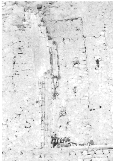
Figure 23: Vaulting tubes in barrel vault, in east wall of frigidarium at Thelepte's baths, Tunisia. Reprinted from R.J.A. Wilson, "Terracotta Vaulting Tubes ( Tubi Fittili ): On Their Origin and Distribution," Journal of Roman Archaeology (1992): 104, fig. 12.
