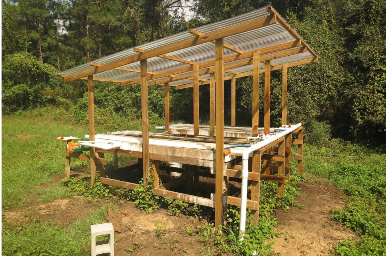
Figure 3.3: Artificial channel system with clear plastic roofing.
