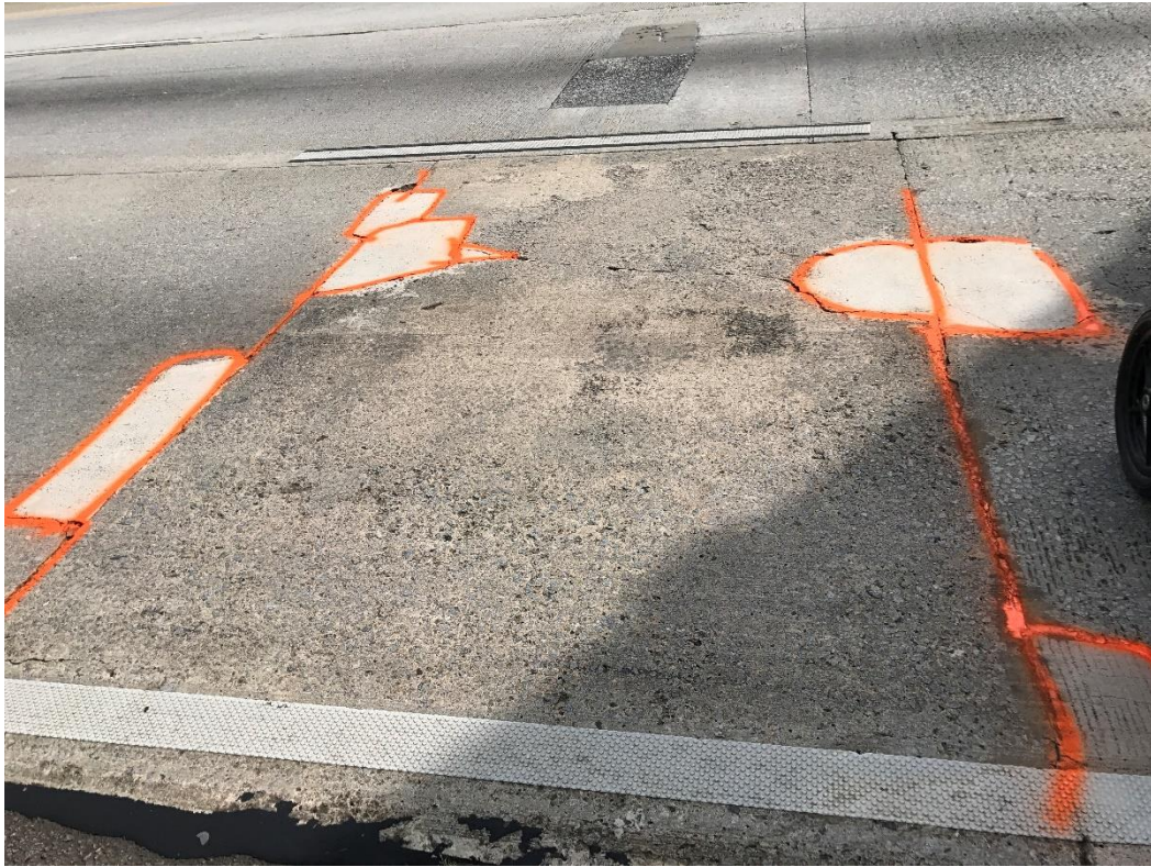
Figure 6.25 – A Patched Area at Outside Lane at S3-d
