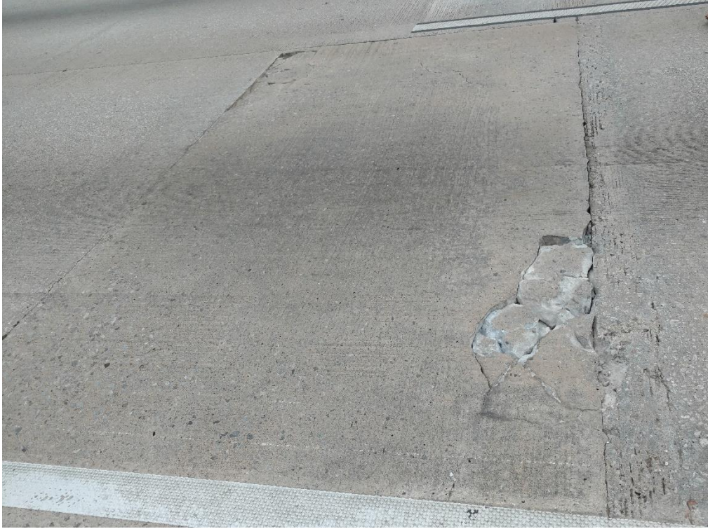
Figure 6.23 – A Patched Area at Outside Lane at S3-b
