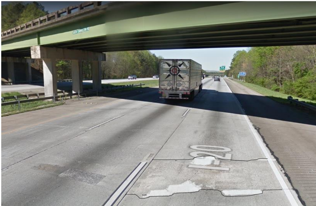
Figure 6.25 – A Patched Area at Outside Lane at S3-d
