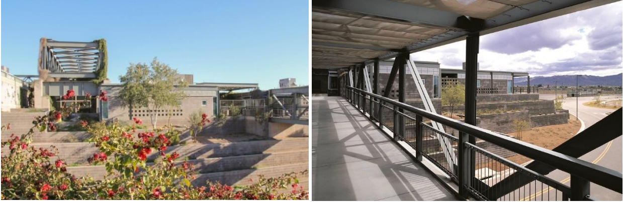
Figure 31: Public entrance and terraced landscape ( Photo by Courtesy of Michael Singer Studio)
