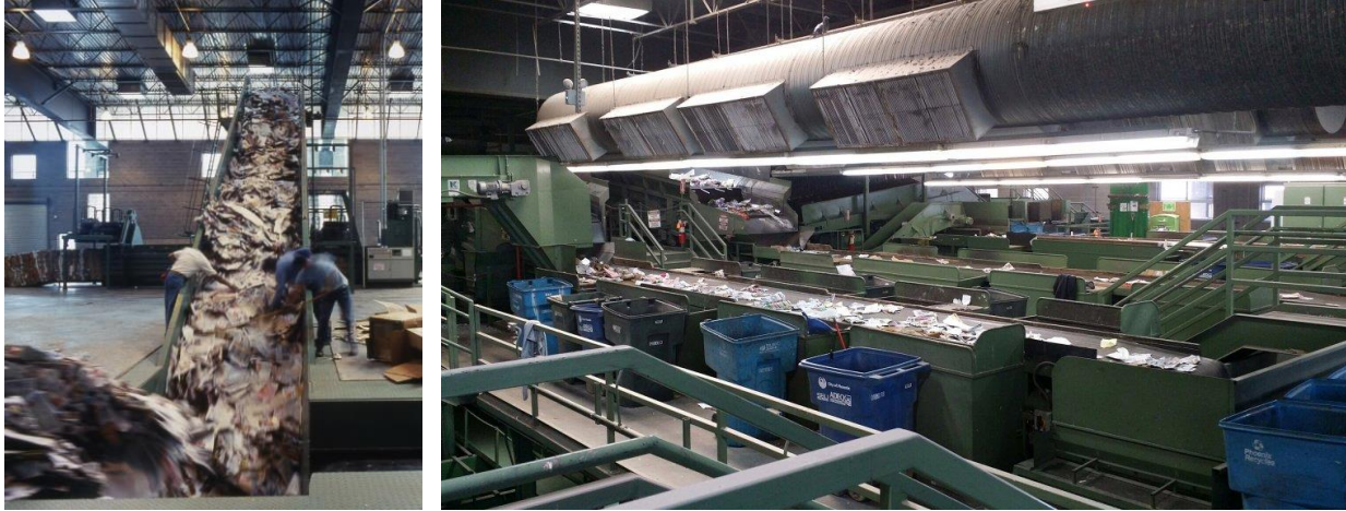
Figure 25: Recyclable materials processing on the first floor of the building
