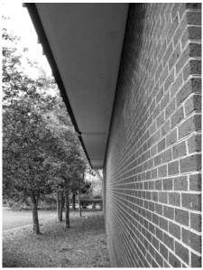
Figure 59. Brick wall and wide roof overhang.
