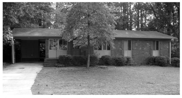
Figure 25. Inline Ranch-type house on Jamagin Drive in Athens, Georgia. Note the horizontal sliding windows and brick pattern.
