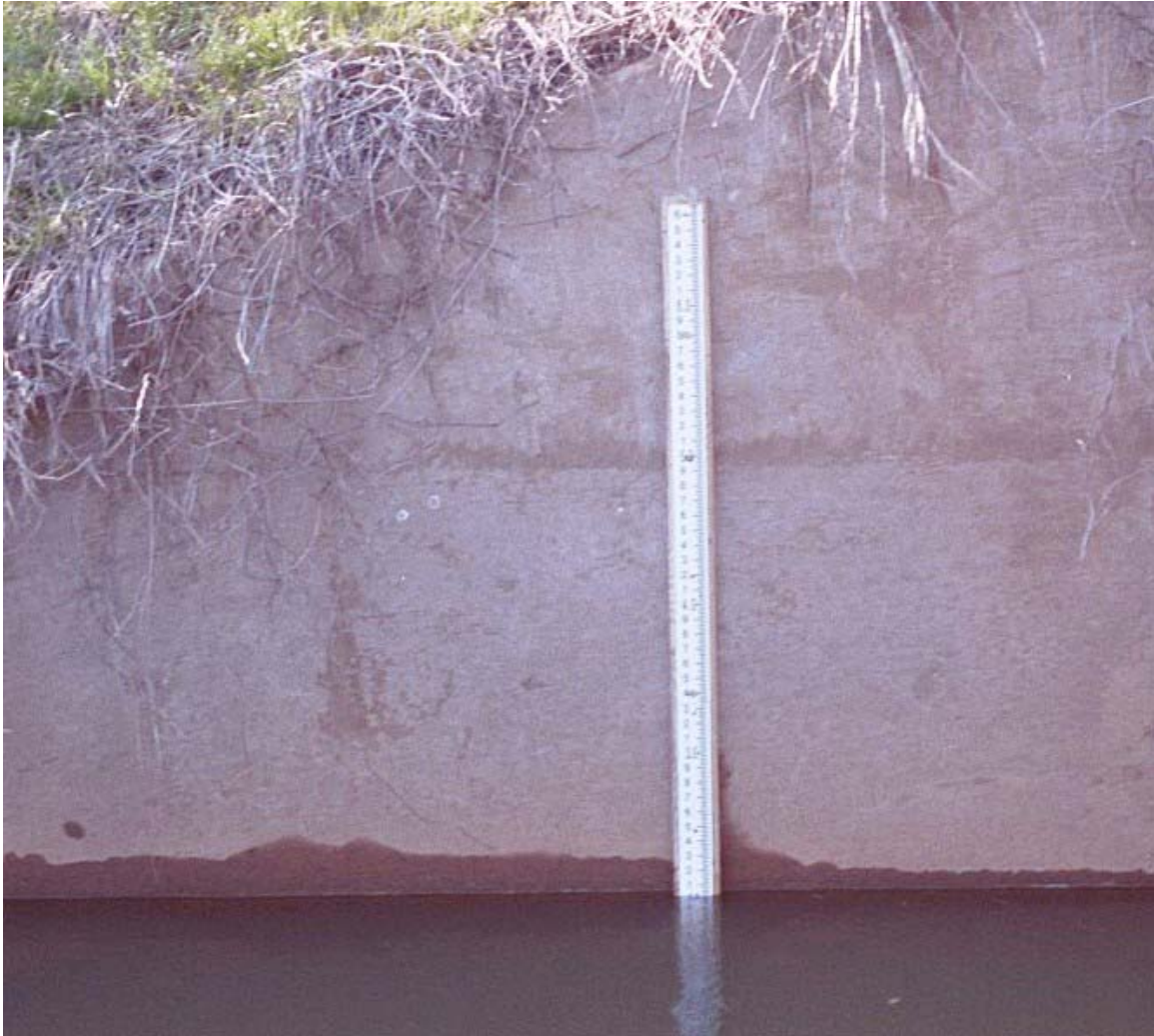
Figure 4.7. Staff gage used for determining flow in East Fork Little River at No Pone Road, attached to the southwest culvert wing wall by the author.
