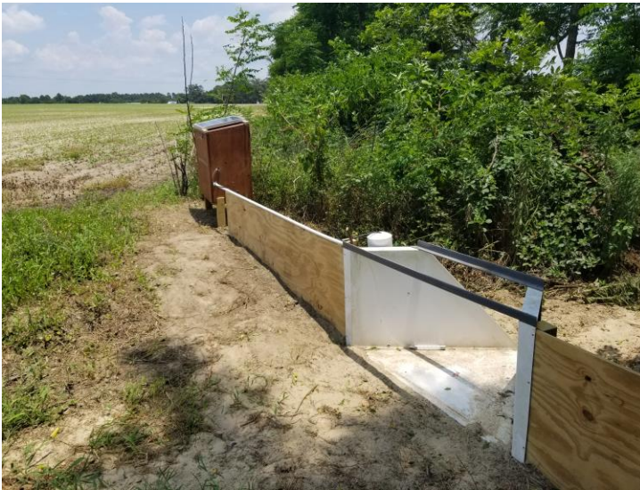
(a) Flume at installation
