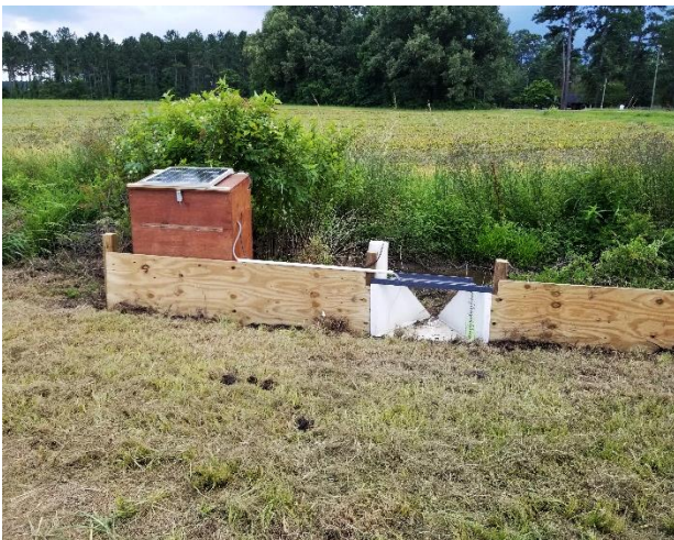
(a) Flume at installation
