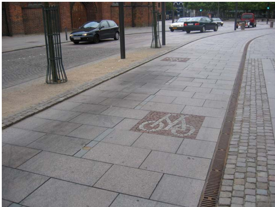
Figure 5.7: Bike lane in central Odense. Bike lanes in the central city blend with the existing historic materials. Note the built in drainage and directional striping inlaid in the stone work. (Photo by author)
