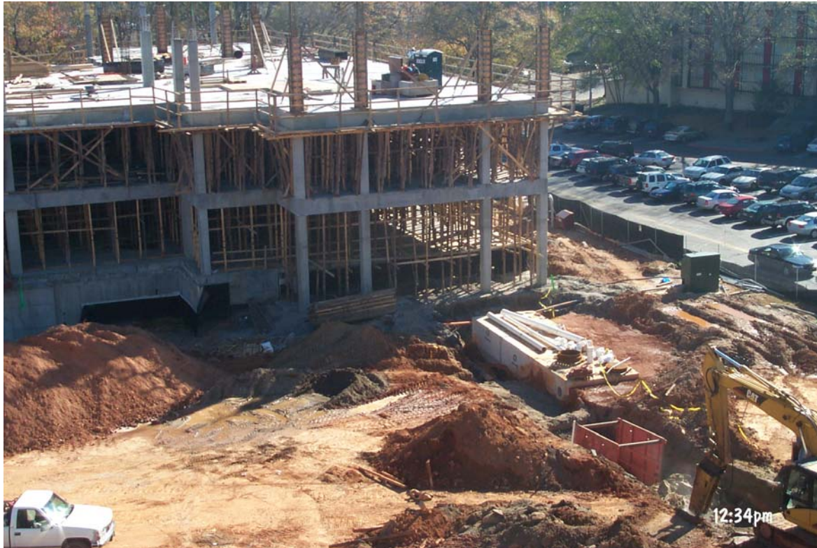
Figure 3.11. Pre-cast concrete cistern set in place, Coverdell Center, University of Georgia
