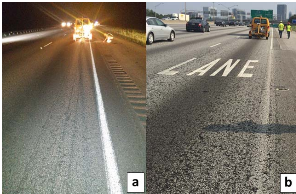
Figure 9.2 - Site Photos (PEM pavements) (a) I-95 (good condition) (b) I-75/I-85 (poor condition)
