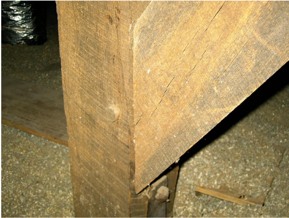
Figure 53: “St. Paul Lutheran Church, Mortis and Tenon Joints
