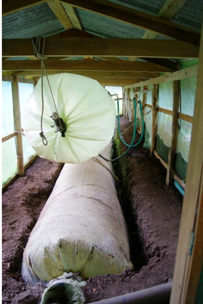
Figure 2.1: View of one of the UGA Costa Rica biodigesters, which served as a model for the thirteen digesters in San Luis.
